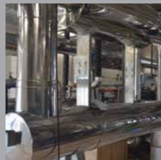
Exhaust Heat Boiler
