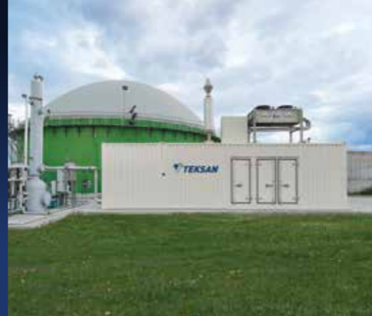
1 x 250 kW Biogas Cogeneration System
