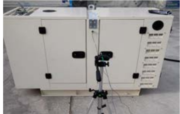
Figure 7: Generator test setup.
